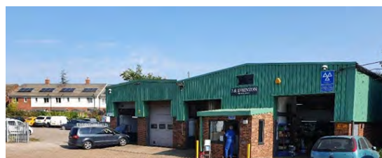
Commercial Unit at the Danbury Business Park.
