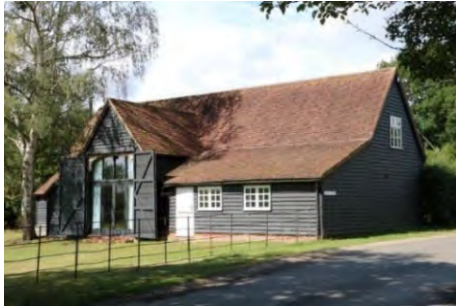
A barn conversion at Gay Bowers repurposing a heritage asset.
